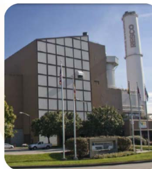
Northeast Maryland Waste Disposal Authority Baltimore "BRESKO" Facility
