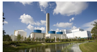
Lee County, FL- Covanta Energy
