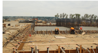
CR&R Eisemann – Perris, CA (under construction)
